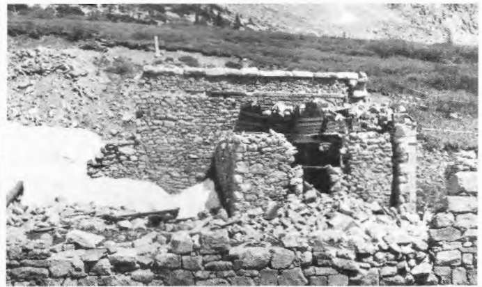
The remains of the engine house at Alpine, Colorado showing the base of the water tank in 1939. Notice the hoops. Photo by Don R. E. Rogers.
