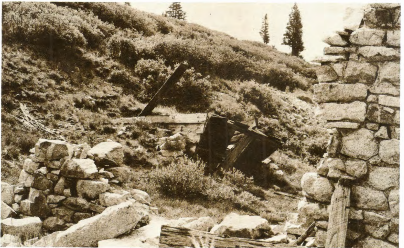
The remains of the Alpine, Colorado, storage shed or "new" section house, just south of the engine house. This building was built right into the side of the mountain.
