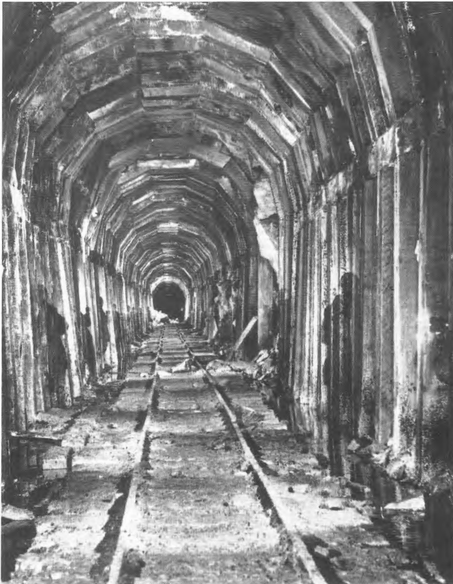
This 1975 photo of the DSP&P Alpine Tunnel shows about 300 feet of the interior from the first big rock fall toward the apex of the tunnel and the east portal beyond.
